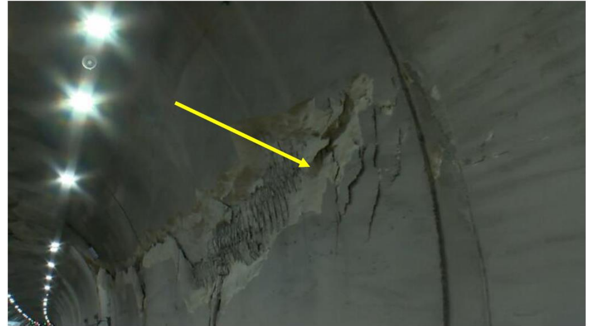
Spalling of concrete linings in Erkenek Tunnel
