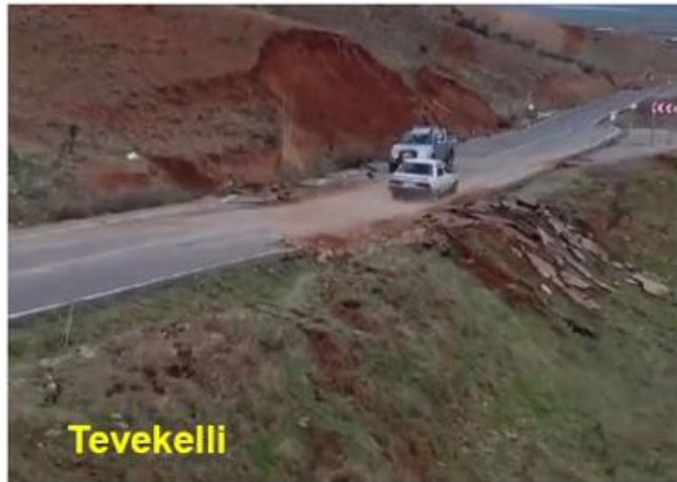
Slope Failures (Land Slides)
