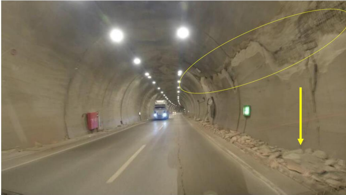
Spalling of concrete linings in Erkenek Tunnel
