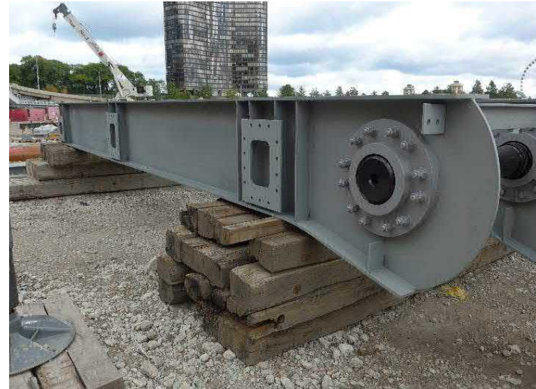
Hinged Sidewalk Girder 2 with end plate moment connection (October 2020)
