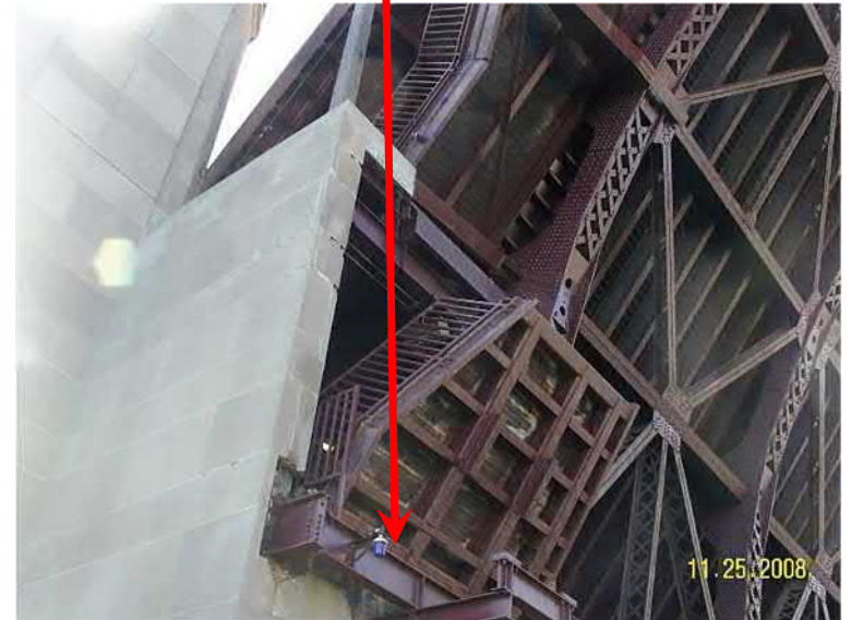
1980s hinged sidewalk, fully-open position, ~75deg
