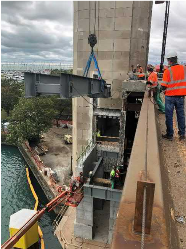
SE Hinged Sidewalk (Girders 1 & 2) being erected
