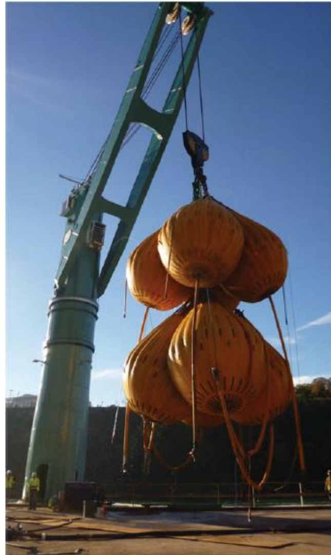
Figure 5: Maid of the Mist Crane Load Test Picture.
