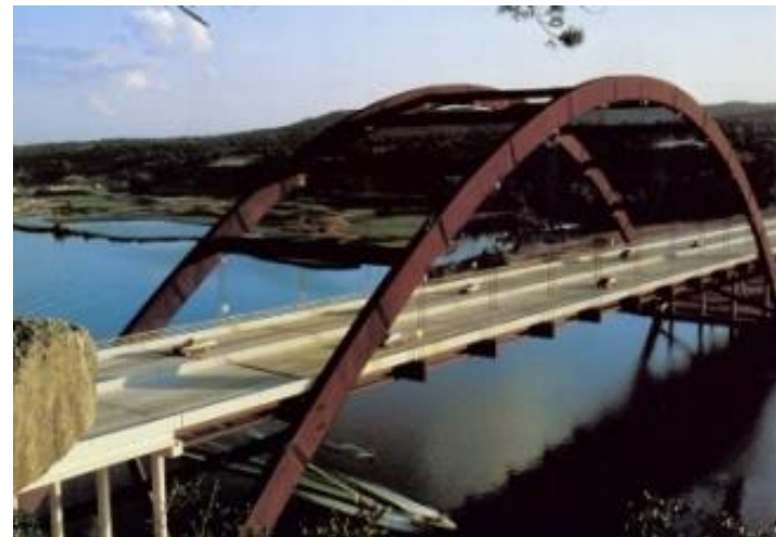
True Arch Bridge (Thrust-arch Bridge)
