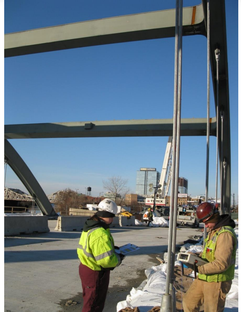
CABLE HANGER: FORCE TESTING
